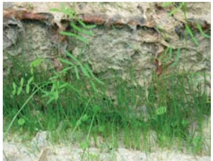
Flexterra and a seed mix were applied to the finished wall.
