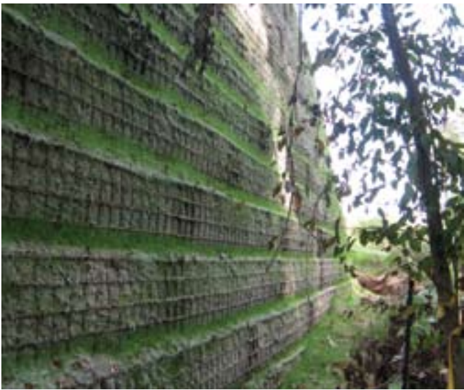
This wall measured 40 feet at its highest point.
